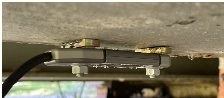
Figure 6.6.2: Strain Sensor Applied to Stringer
