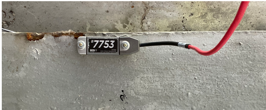
Figure 6.6.1: Strain Sensor Applied to Stringer
