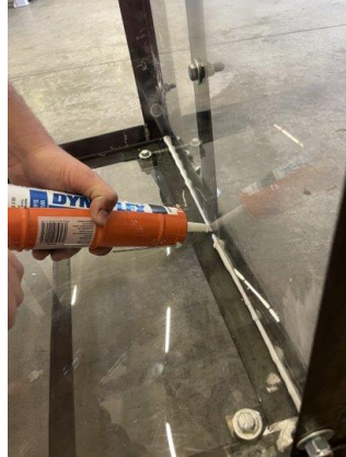
Figure 22: Caulking the Flume
