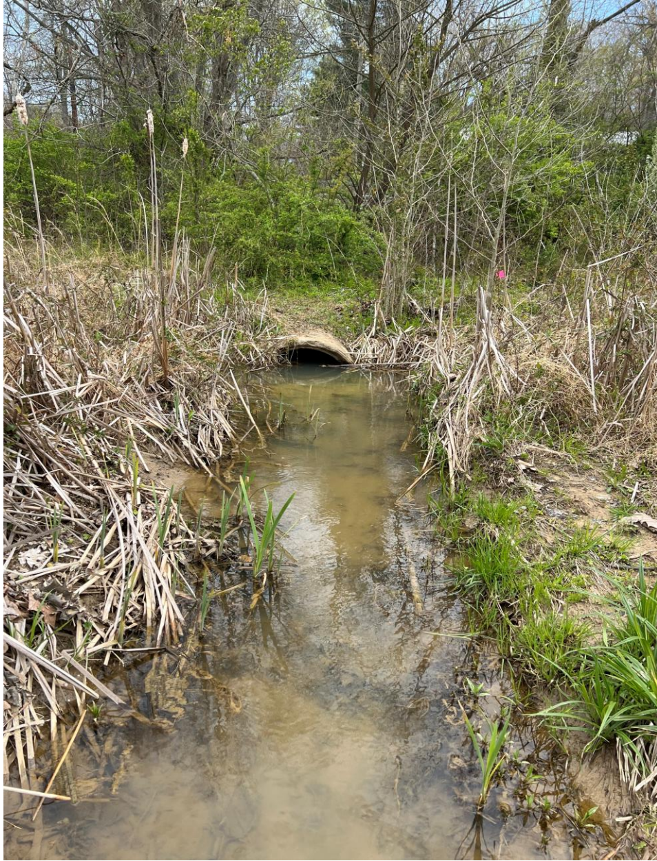
Figure 1716. Downstream of Farm Culvert
