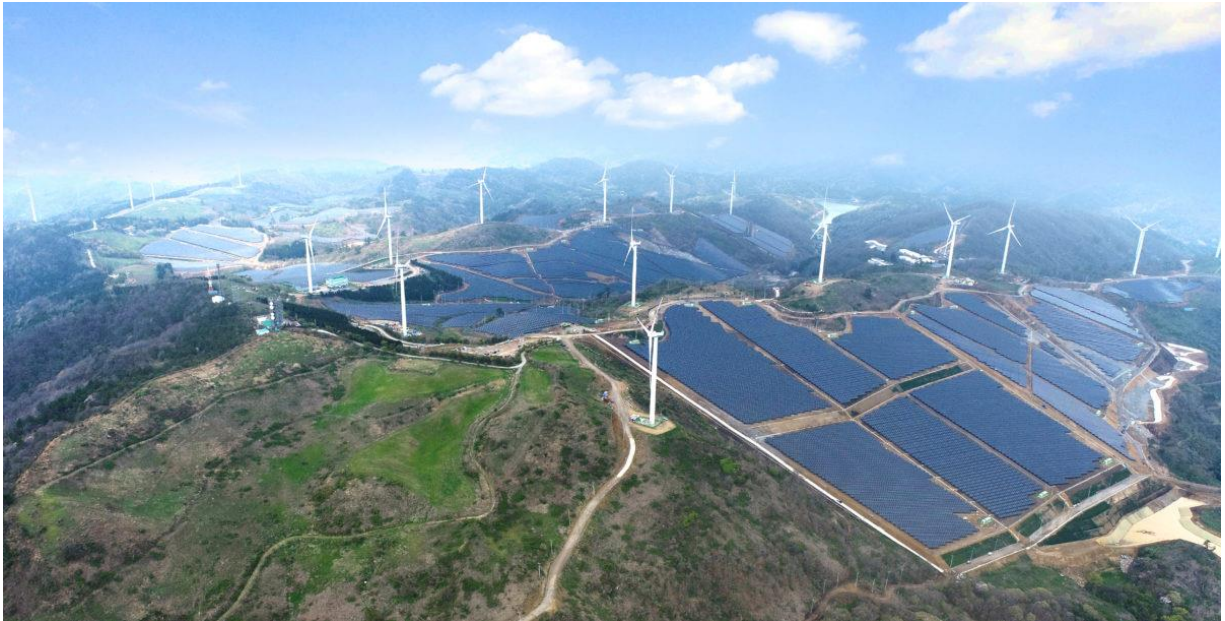
Figure 15: Aerial View of JA Solar Wind / Solar Farm, South Korea [12]
