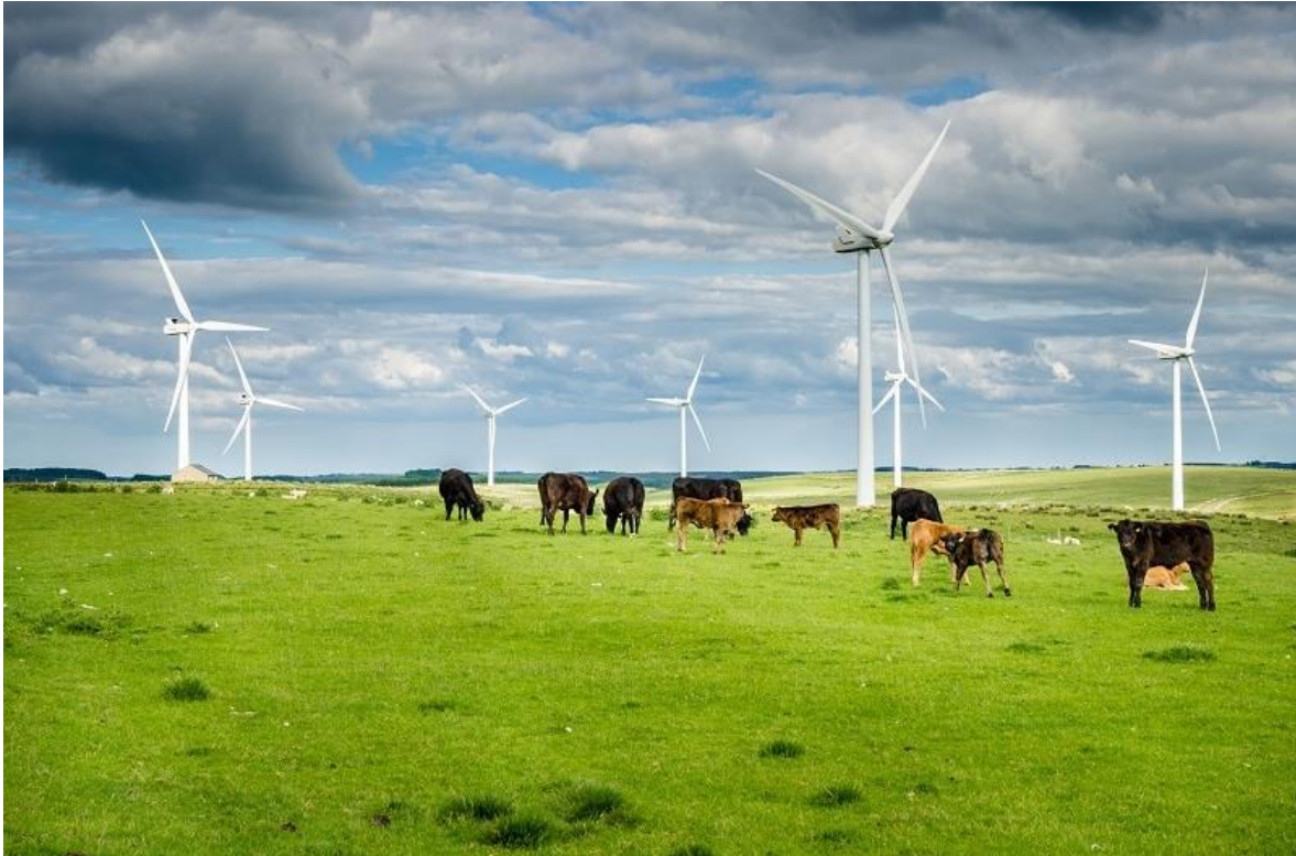
Figure 5: Wind Farm with Alternative Ground Use [22]
