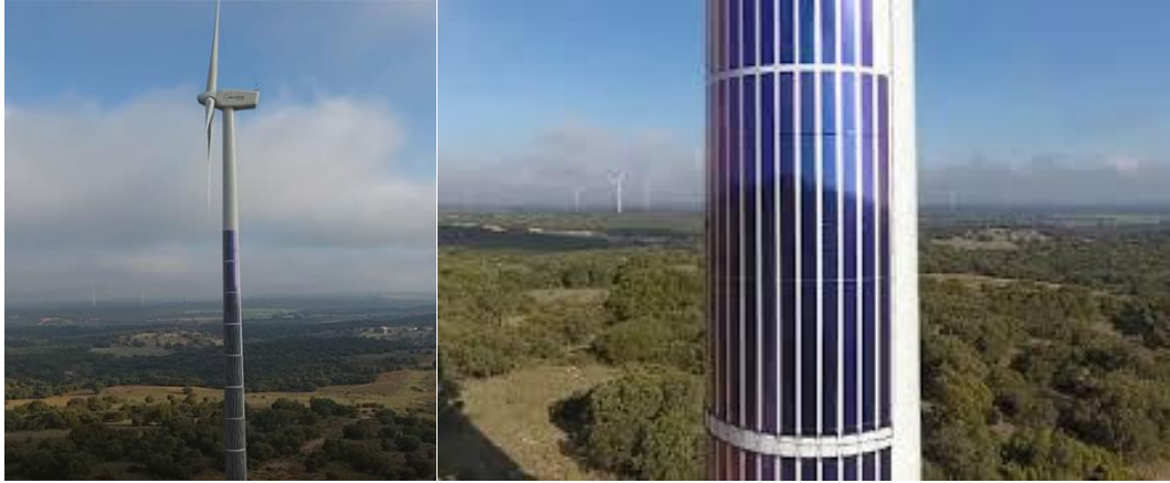
Figure 17: Acconia Wind Turbine with Flexible Solar Panels [3]
