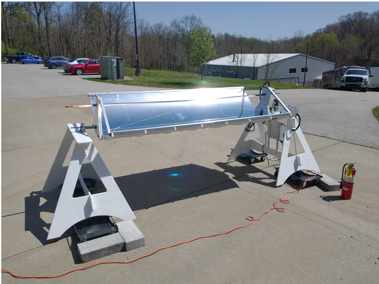
Figure 1: Final implementation of parabolic trough concentrated solar system
