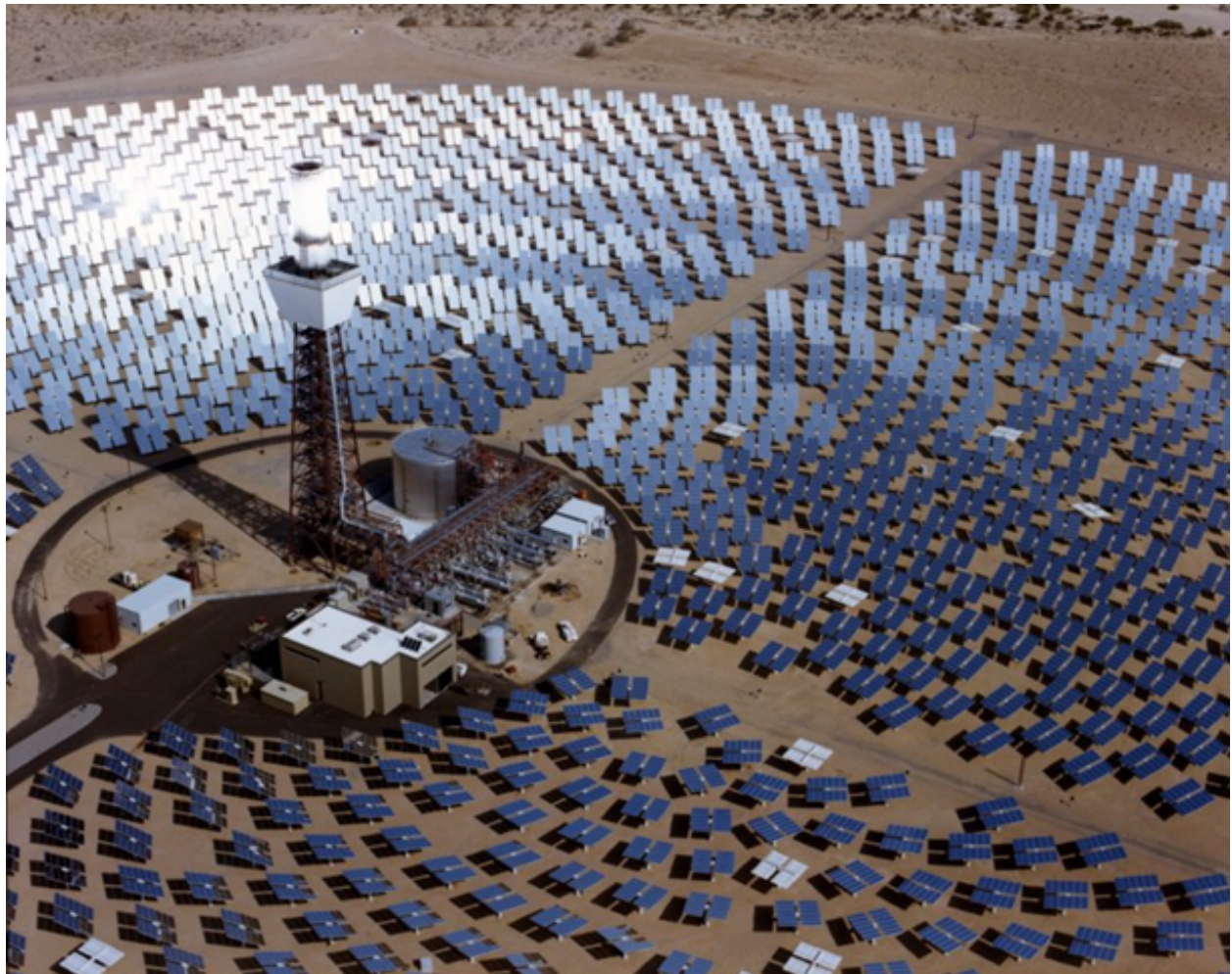
Figure 2: Example central tower CSP system [1]
