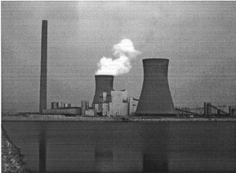
Figure 1. Rockport Power Plant.
