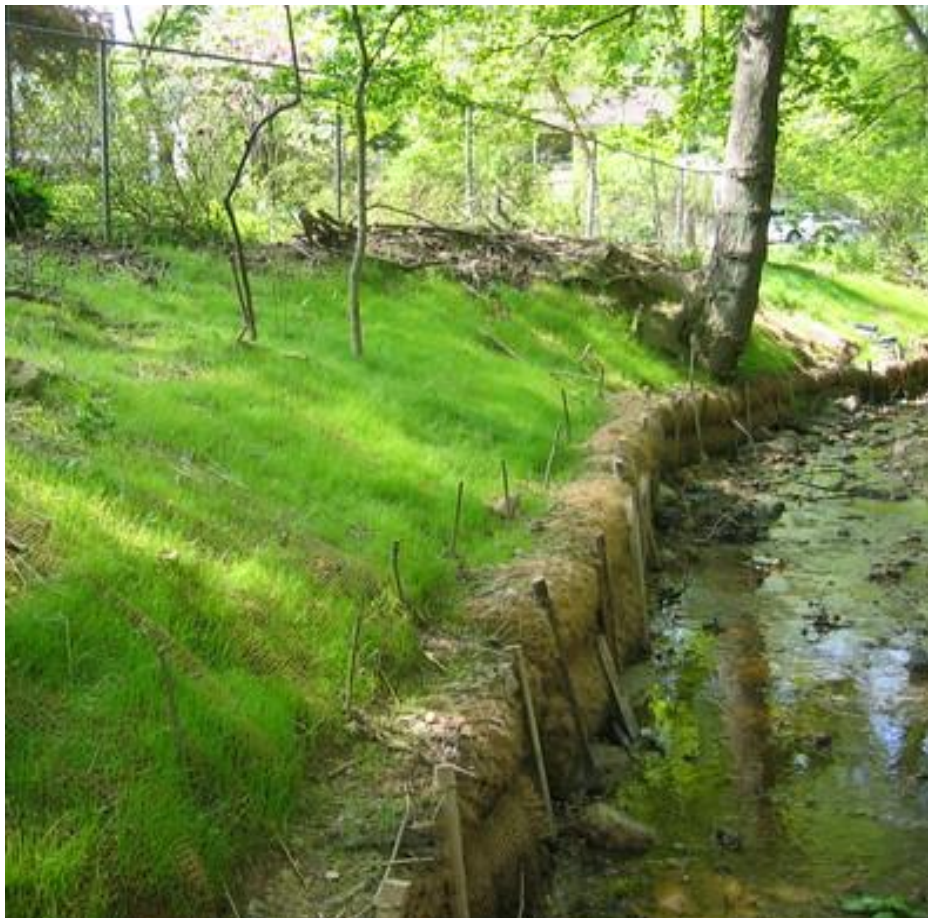
Figure 11: Fresh Installation of a Vegetated Soil Lift
