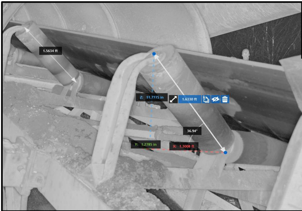
Figure 10: FARO Scan of Conveyor Rollers
