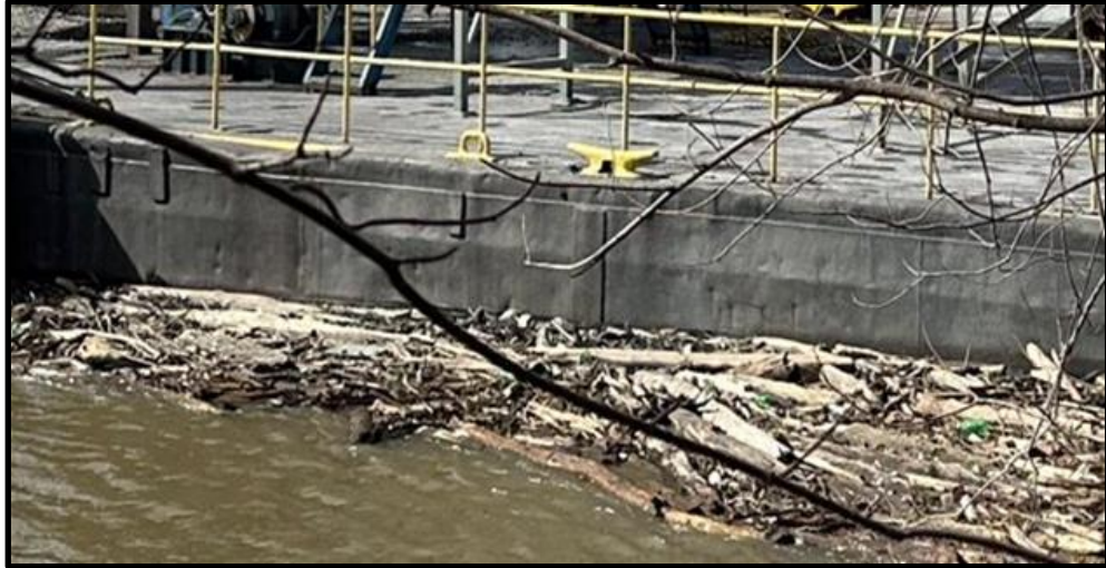
Figure 12: Build Up of Driftwood Around Dock Barge
