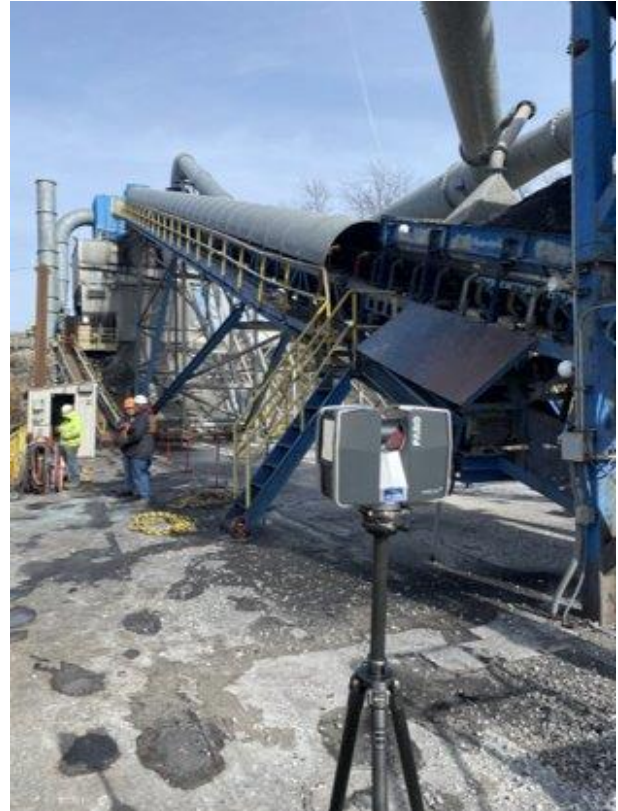
Figure 24: FARO Scanner in Use at Project Site
