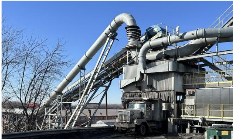
Figure 18: Trucks Being Loaded from Figure 22 Conveyor
