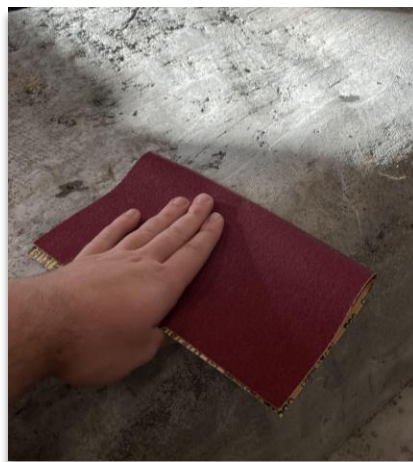
Figure 18. Hand Sanding Rough Patches.
