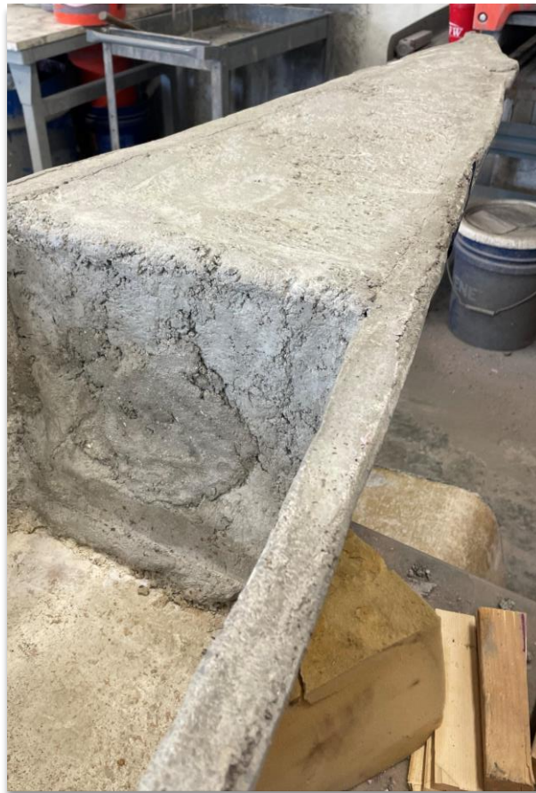
Figure 19. End Caps Post-Pour Before Sealant and Sanding.
