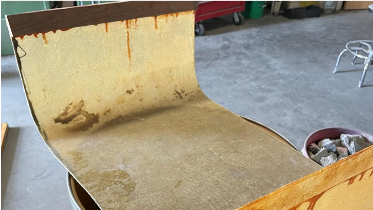
Figure 9. Removed Fiberglass Cross Section.
