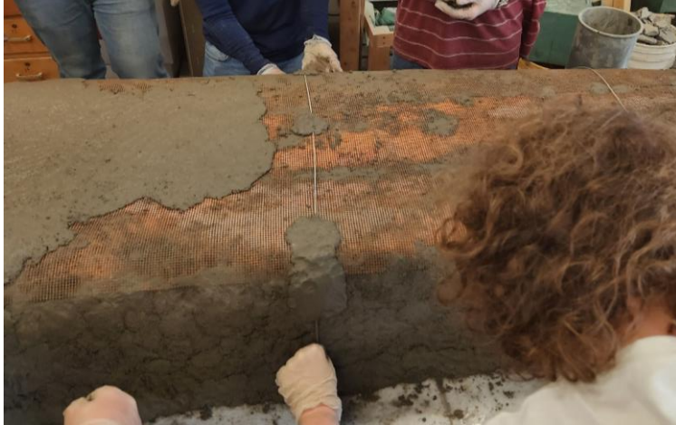
Figure 16. Application of Reinforcement.
