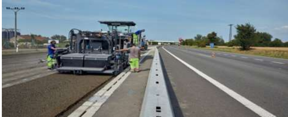
Figure 20: Cement Treated Permeable Base
