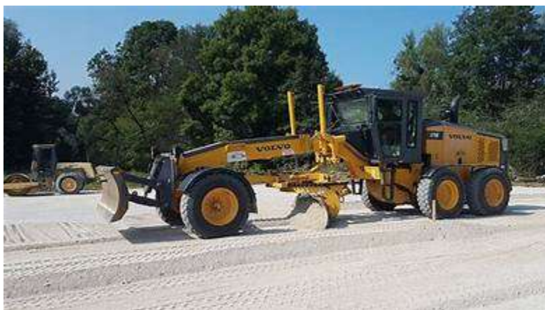
Figure 18: Motorgrader for Crushed Aggregate Grading
