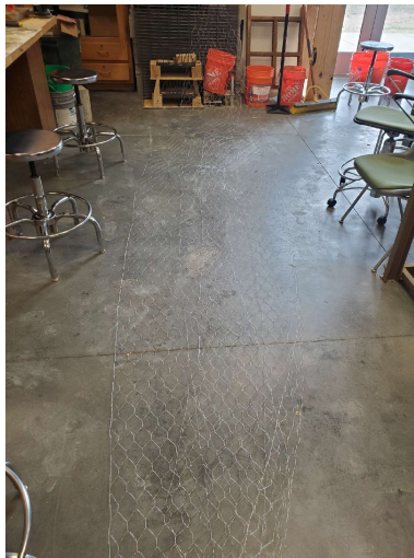
Figure 13: Chicken Wire Reinforcement
