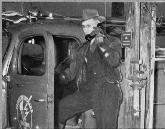
Mobile two-way telephone equipment on trucks and cars keeps service and operating forces in constant contact with headquarters, speeds up service, helps meet emergencies.
