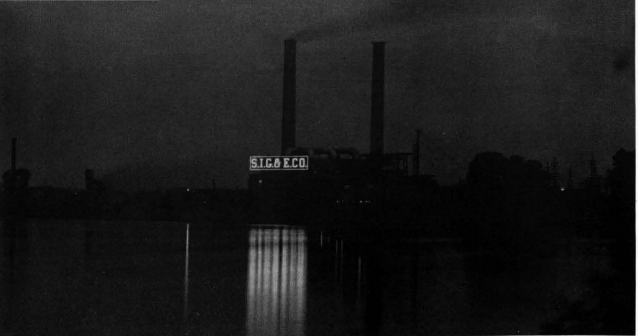
Ohio River Generating Station, Evansville
