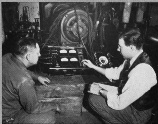
Company representative operating an electric motor analyzer to check motor performance for customer, and improve service.
