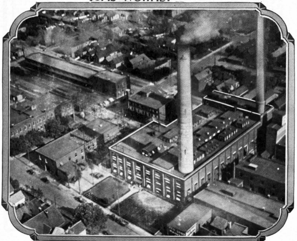
DIVISION ST. ELECTRIC STATION
