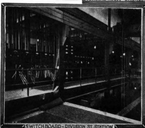
SWITCHBOARD - DIVISION ST. STATION
