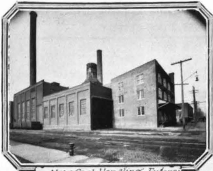
New Coal Handling Extension Rear. Division St. Station.
