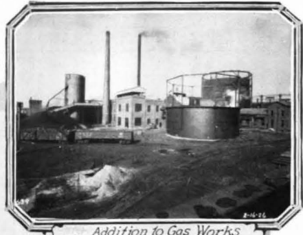
Addition to Gas Works To House Water Gas Set. New Gas Holder.
