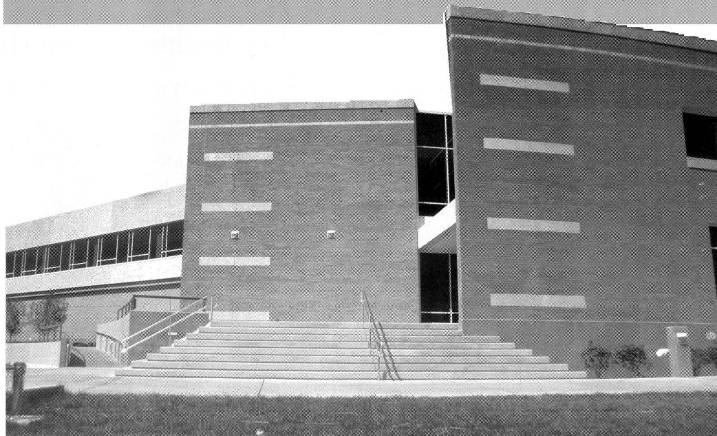
A new entrance on the south side of the University Center enhances the sweeping arc of the addition.
