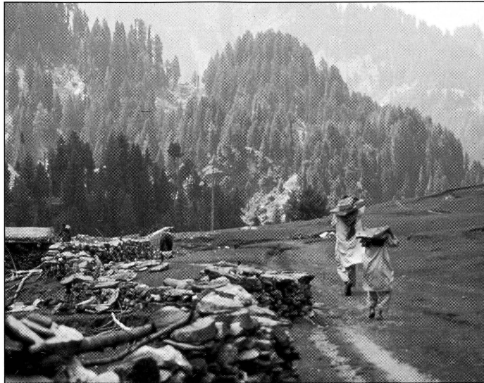
Villagers on Gat Kandao (Gat Pass) construct a rock wall.
