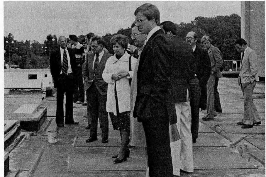
ISU Board of Trustees members visited the site of the new Health, Physical Education and Recreation building during their October Board meeting on the ISUE Campus.
