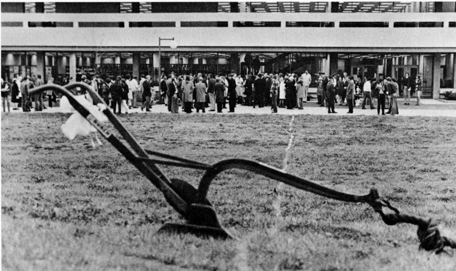
With muscle furnished by the audience, an old-fashioned plow, donated by Burch Plow Works of Evansville, was used to turn the first dirt for the University Center.
