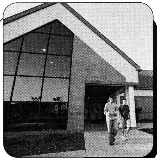
Residence Life Office
