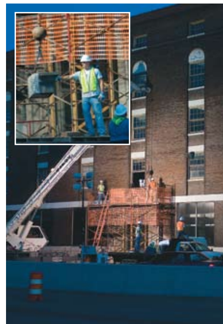
The archway at Orr Iron Company was removed before demolition of the building and will have a new home in the University Center's addition.
