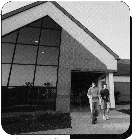
Residence Life Office
