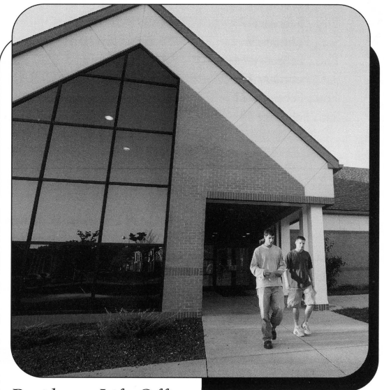
Residence Life Office
