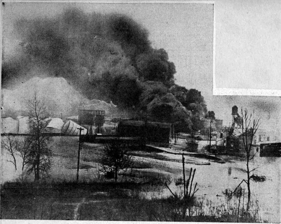
After the flood—fire! To the terror of water gone mad is added the horror of flame rampant. Blazing oil from tanks that exploded at Cincinnati spreads out on the resistless current and touches building after building. Observe two of the overturned tanks. An area three and one-half miles long and a half mile wide was swept by the fires. (International News Sound photo.)
