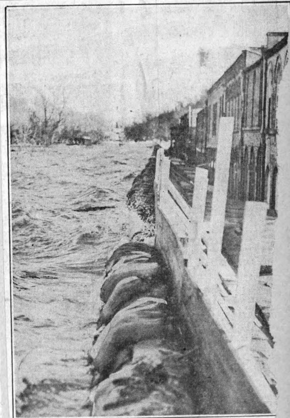
ONLY SANDBAGS HOLD THE RIVER BACK The Mississippi lashing against sea wall at Hickman, one of major danger points in flood zone. The river is above the top of concrete levee protecting the
