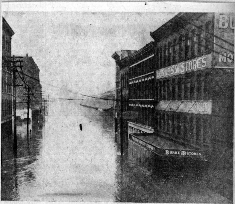
Water at the 65.4-foot stage has caused a complete suspension of business in the W. Front st. wholesale and warehouse section in Cincinnati. Note the great height of the flood. (International News photo.)
