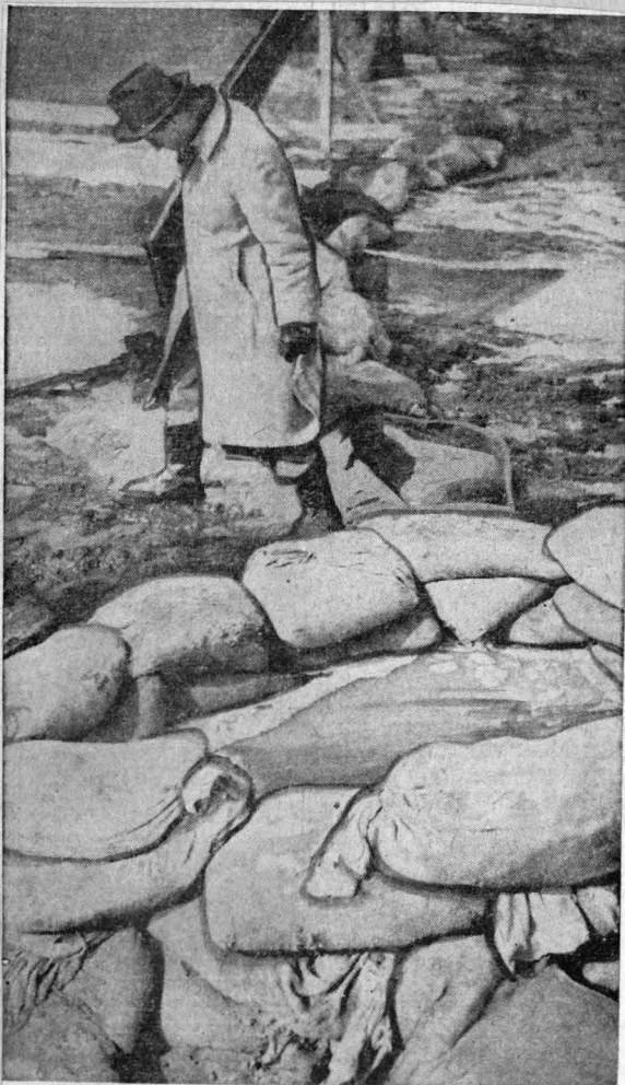
BELOW EARTH FLOODS COME TO SURFACE A government engineer examines a "sand boil" in a Cairo street. The phenomenon is caused by floodwaters forcing their way up through the ground. The Ohio, at a 59.7-foot level, is lapping at the sandbags atop the levee. [Daily News-Wide World photo.]
