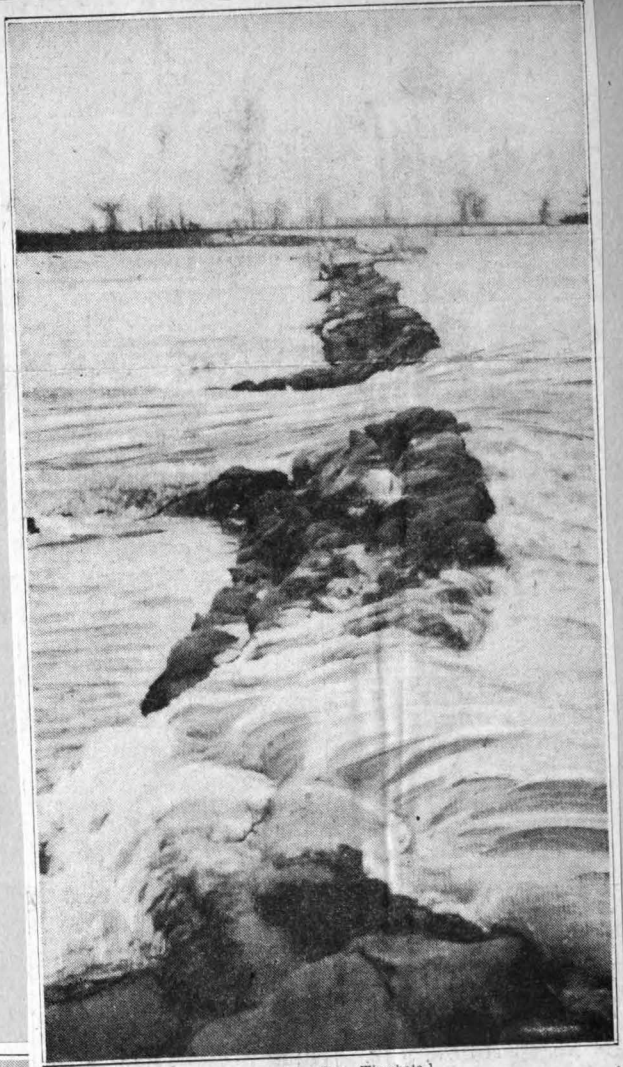
MISSISSIPPI TEARS HOLE IN DIKE —Twenty foot gap in Slough Landing neck dike, a secondary levee at Bessie, Tenn., as waters rushed out over 20,000 acres of land. The area was already partially inundated and may become a new channel for the raging river.
