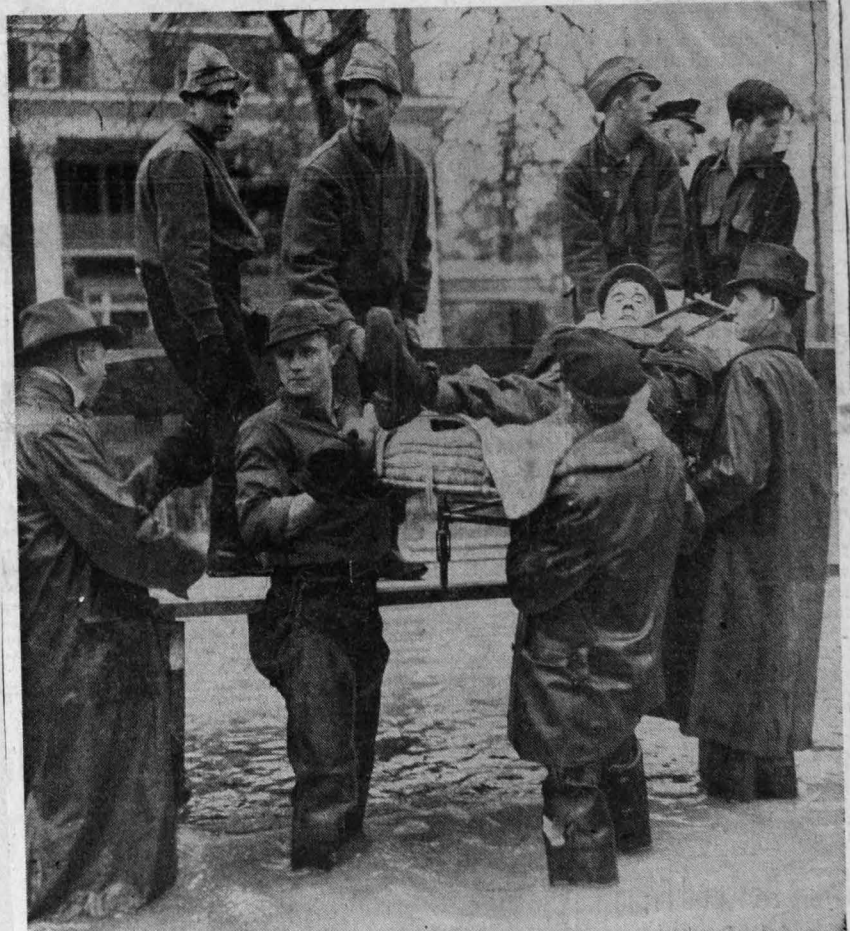
Bed-ridden flood victim being removed by relief workers from inundated home in Paducah, Ky., as other members of family, which braved privation and death
