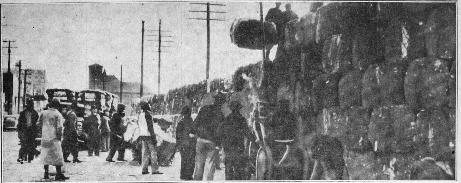
MEMPHIS BOLSTERS MISSISSIPPI RIVER LEVEE WITH BALES OF COTTON —Workers in Tennessee city erect an expensive wall to hold back waters of rising stream, using bales of cotton worth $60 each to reinforce dike. This picture was made yesterday on Front street as 25,000 huge bundles were hoisted into place. The city prepared to care for 50,000 expected refugees. Many flood victims already there were transferred to make room for thousands of others who will flow in if the levees give way. [Associated Press Wirephoto.]
