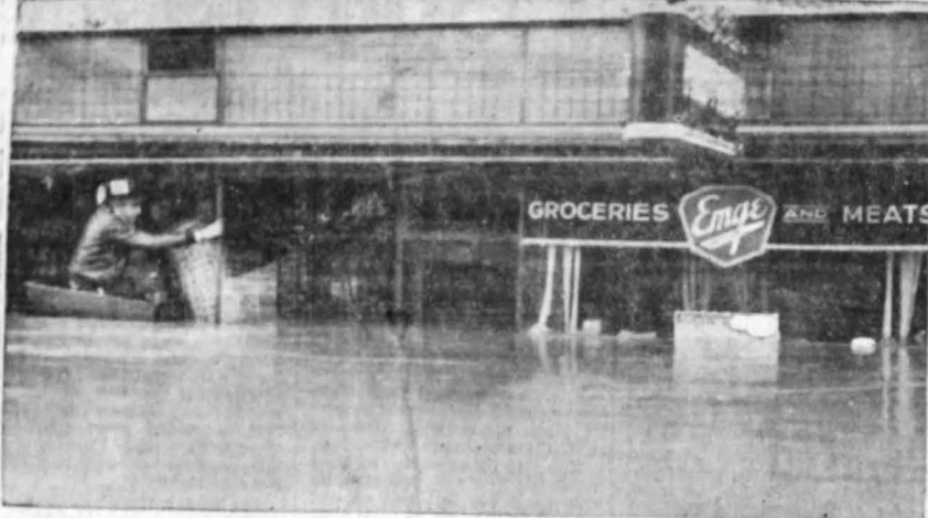
The Emges never dreamed they would enter their grocery store on Kentucky Avenue in a row boat . . . but here they are as they stretched chicken wire on the inside to keep the groceries on the inside looking out. The force of the water has broken one of the windows.
