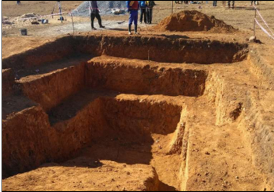
Figure 2.2.2 Example of Benched Excavation
