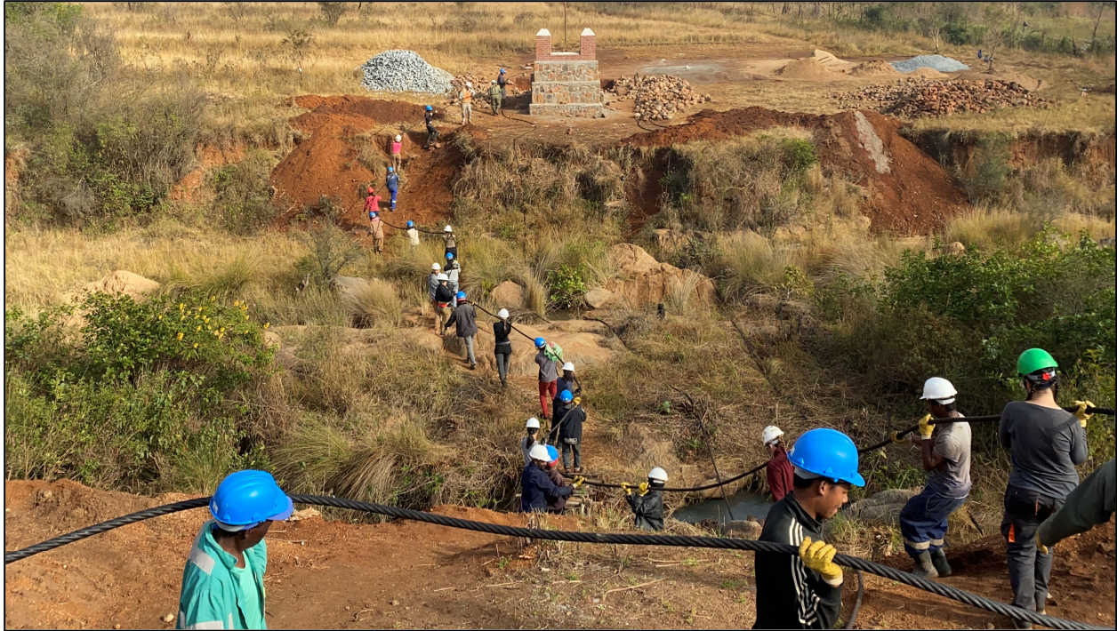
Figure 5.1.1 Bringing Cables to Site
